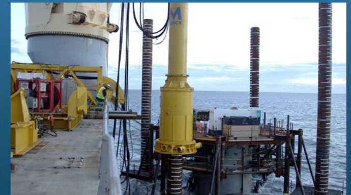
ADDITIONAL PILES SECURING MONOPOD
