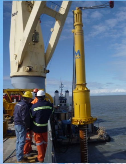
PRE-PILING OF KING PILE
