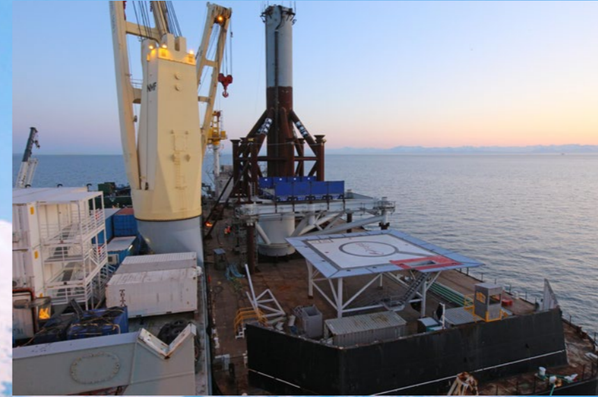
MONOPOD DELIVERY BY BARGE
